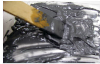
Figure 10: Mix the two components of the epoxy.
